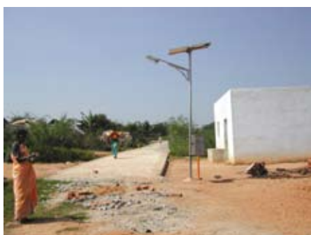
A photovoltaic street light
