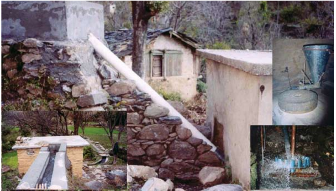
An improved water mill of IIT Roorkee design
